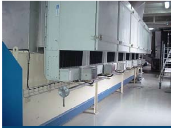
2 passages cooler fitted with filters
